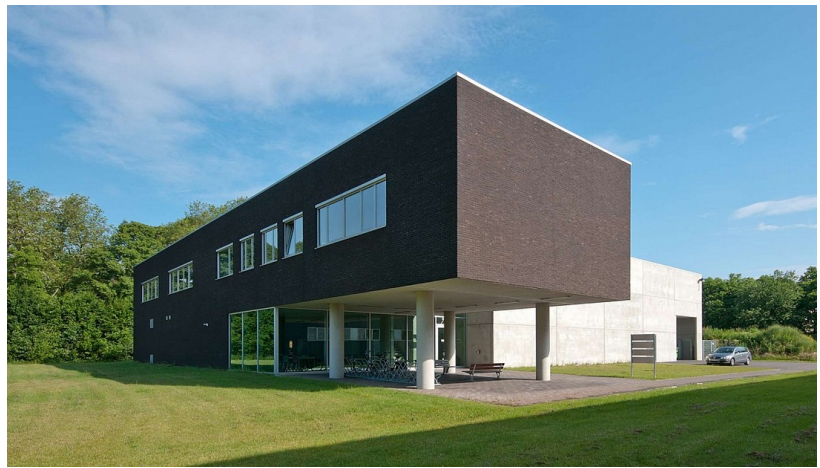
Construction of a welding center institute
