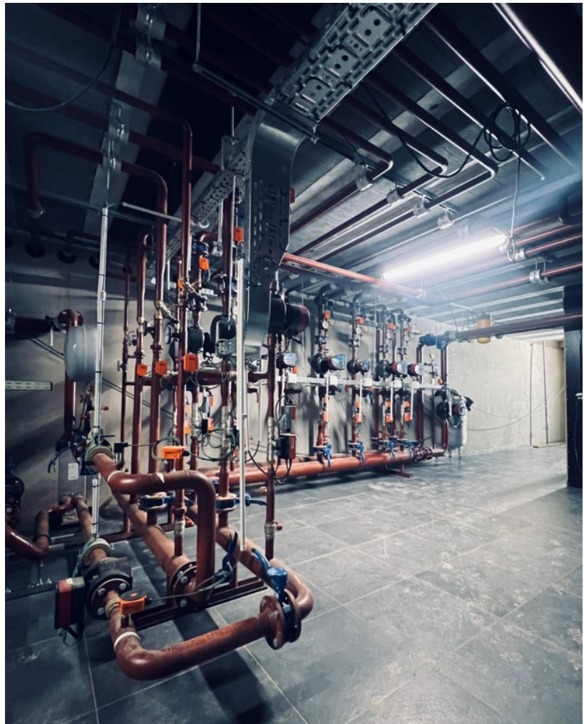
HVAC and plumbing package, private project renovation.
