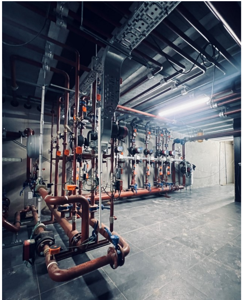
HVAC and plumbing package, private project renovation.
