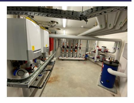
HVAC and SANITARY Renovation of listed building Heat production gas-fired boilers Cold production with monoblock chiller Ventiloconvectors 2 Air handling units for cooling and heating with electric steam humidifier and dehumidification.
