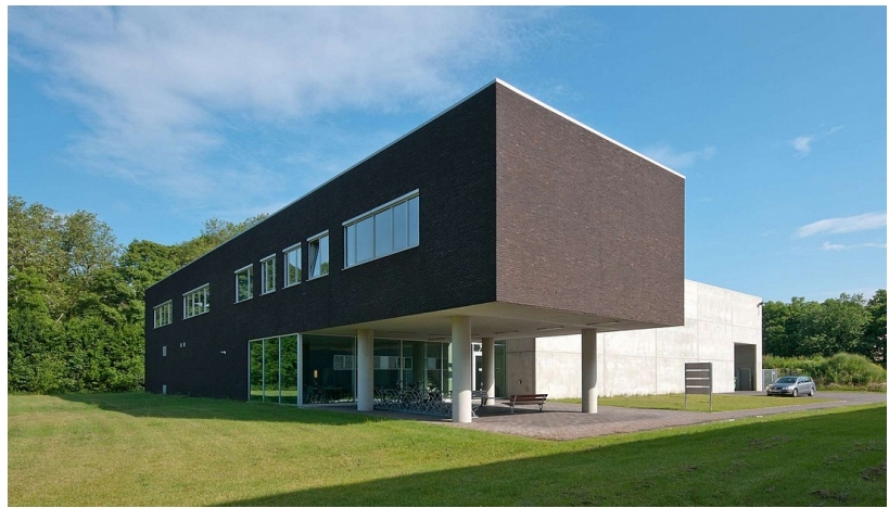
Construction of a welding center institute
