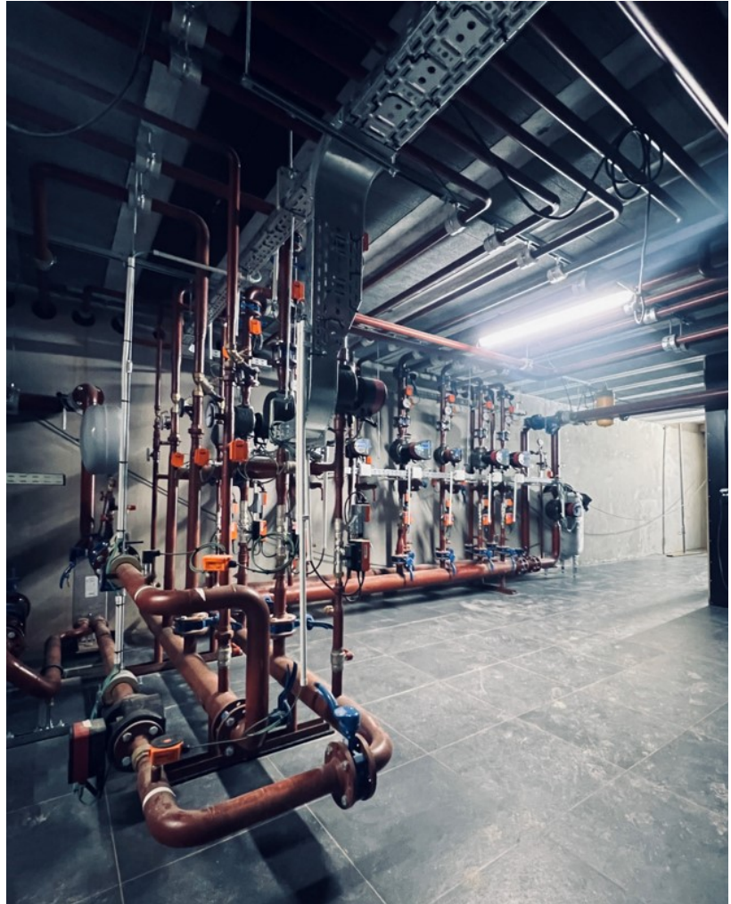
HVAC and plumbing package, private project renovation.
